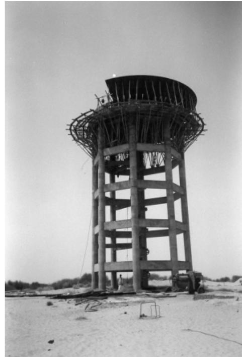
**Figure 4.** A new Elevated Service Reservoir under construction. For scale, note the man standing under it. (Author photo)
