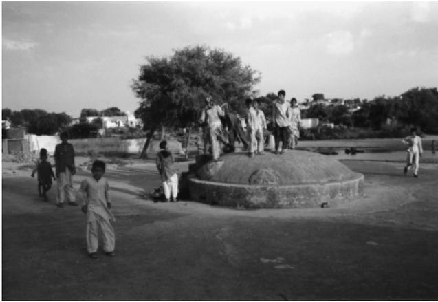
**Figure 2.** A passive rainwater harvesting system called a *kund*. Rain that falls on the surrounding surface area drains toward the ground-level holes in the dome and into a tank below. The girls are drawing water out with a bucket on a rope and then filling their pots. (Author photo)
